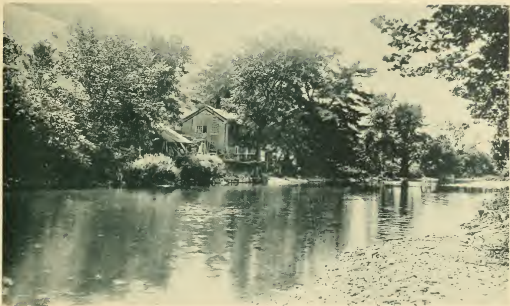
VIEW NEAR RED BRIDGE—LOOKING SOUTH.
